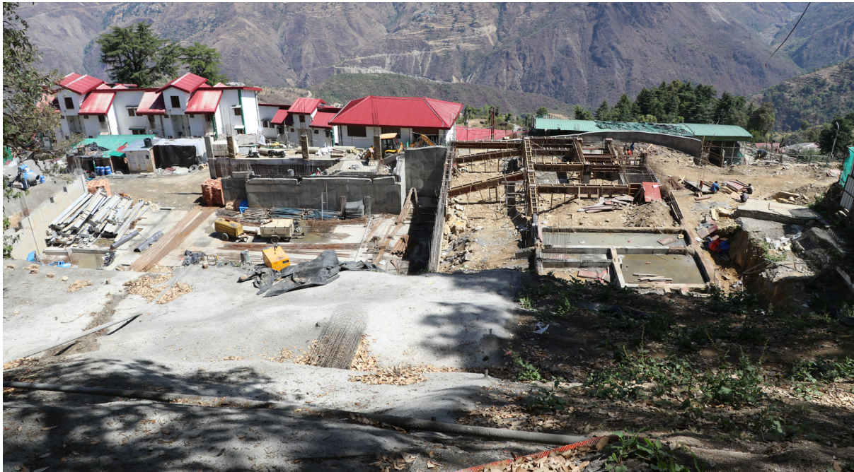
Figure 1.18: C/o new auditorium at old horse line
