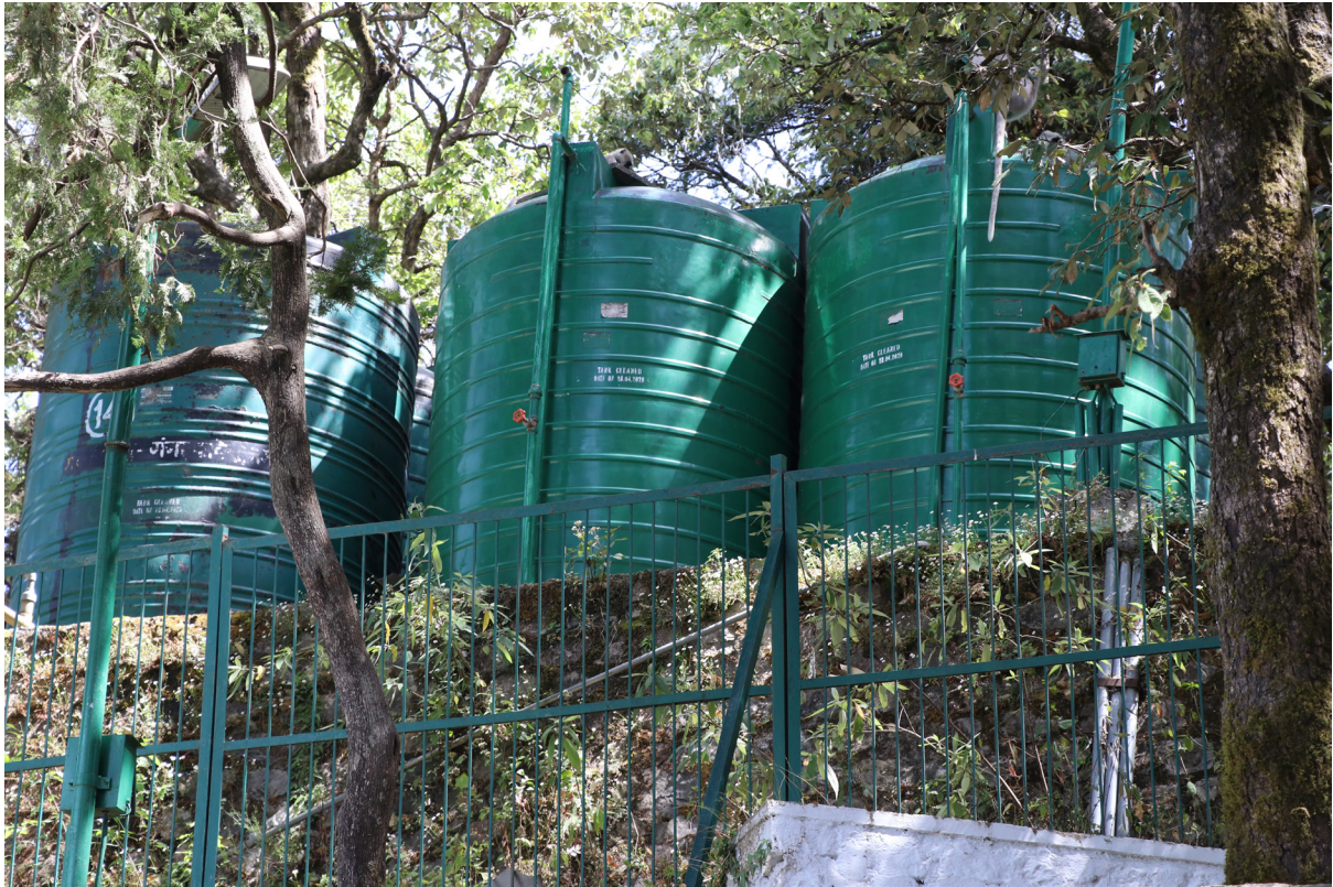
Figure 1.8: Water storage tanks
