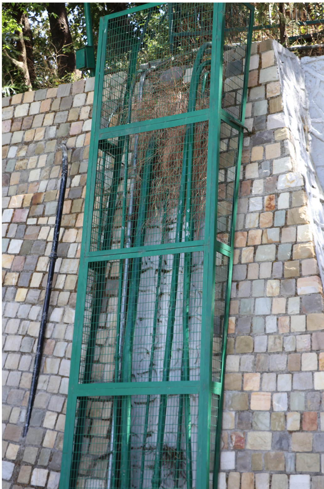
Figure 1.7: Electrical wiring and pipeline assembly
