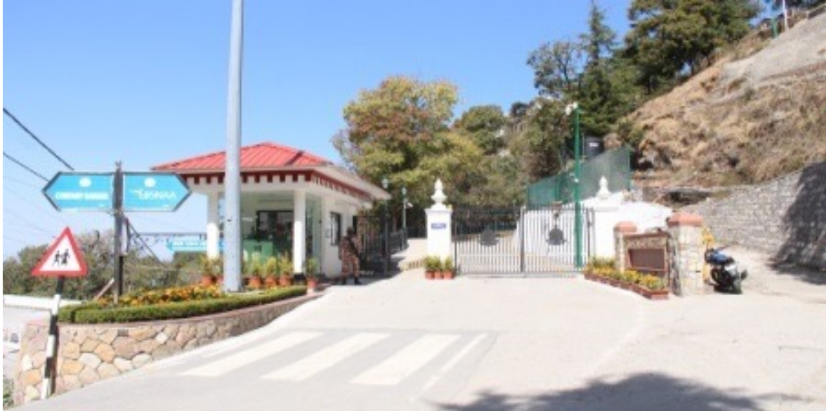
Figure 1.14: Reconstructed main entrance
