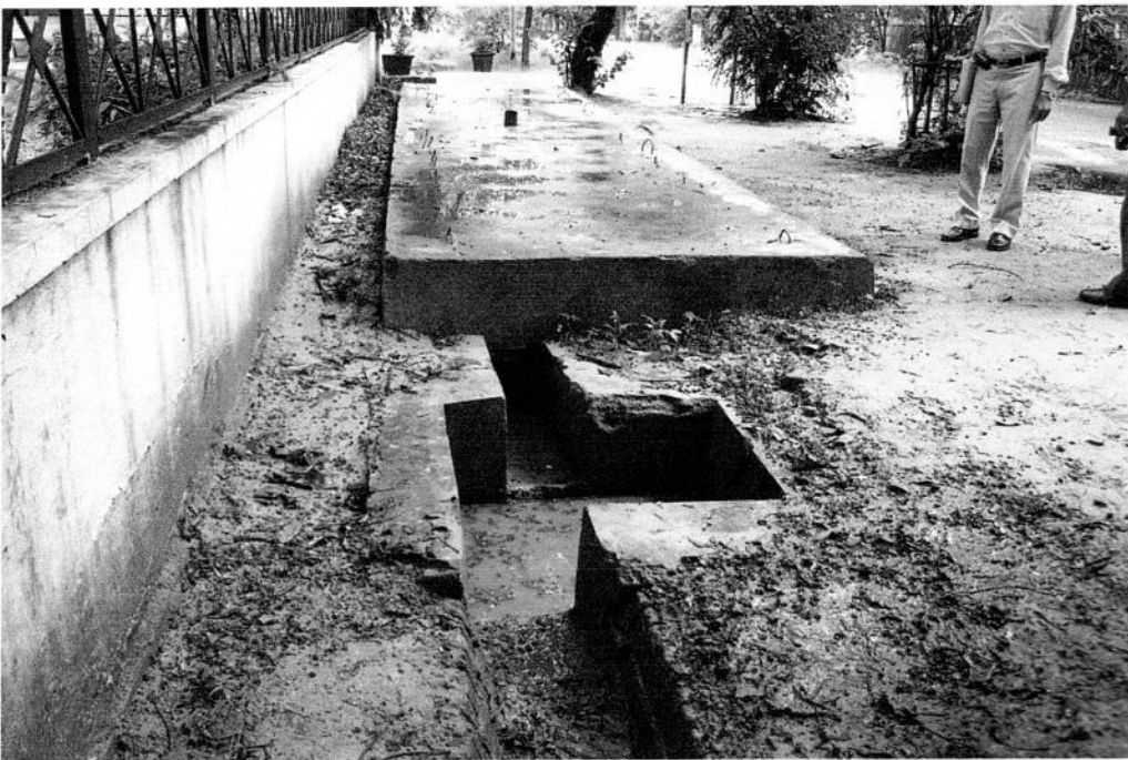
Fig 5.6 RWH by Trench with Bore method at S.P. Marg Officers Colony
