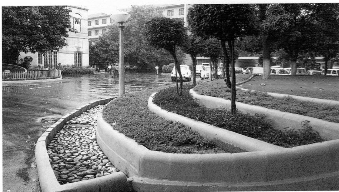
Fig 5.4 RWH by Trench method at Baroda House
