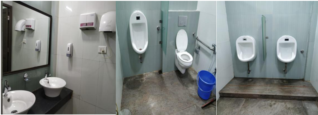
Photograph 29: PT at Triveni Shopping Complex (Internal)
