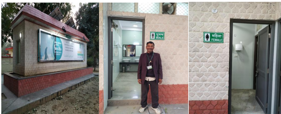
Photograph 28: PT at Triveni Shopping Complex (External)
