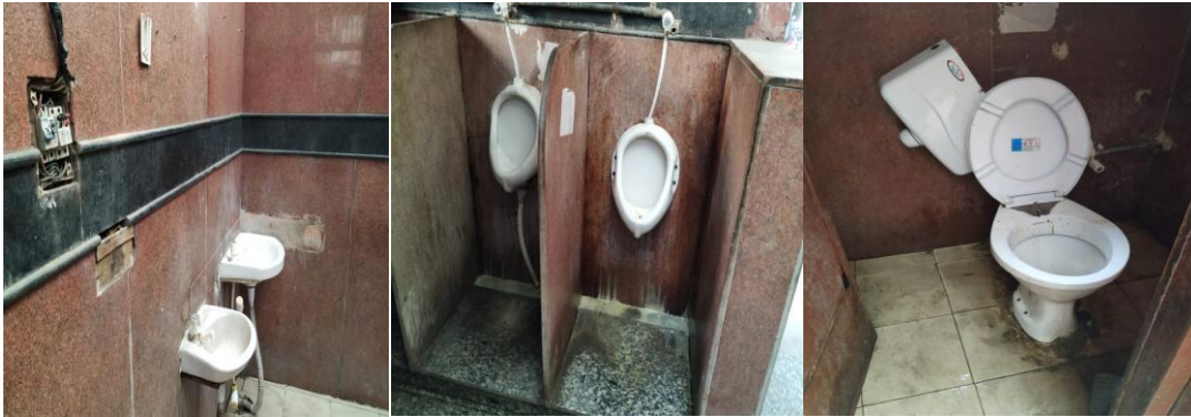
Photograph 23: Old PT at Shastri Bazaar (Internal)
