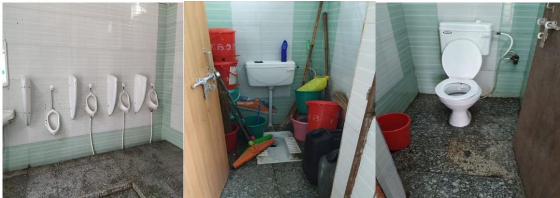
Photograph 27: PT at Shri Nagesh Garden (Internal)
