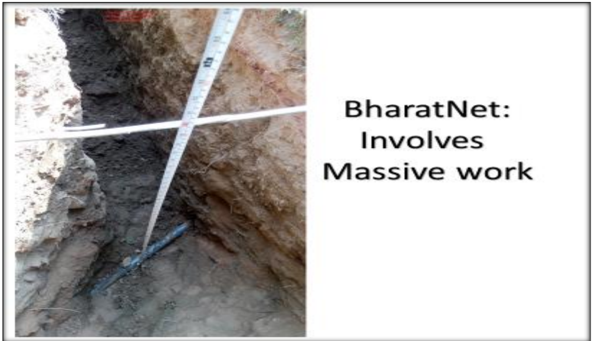
Fig 18 :Bharatnet Cable Laying work
