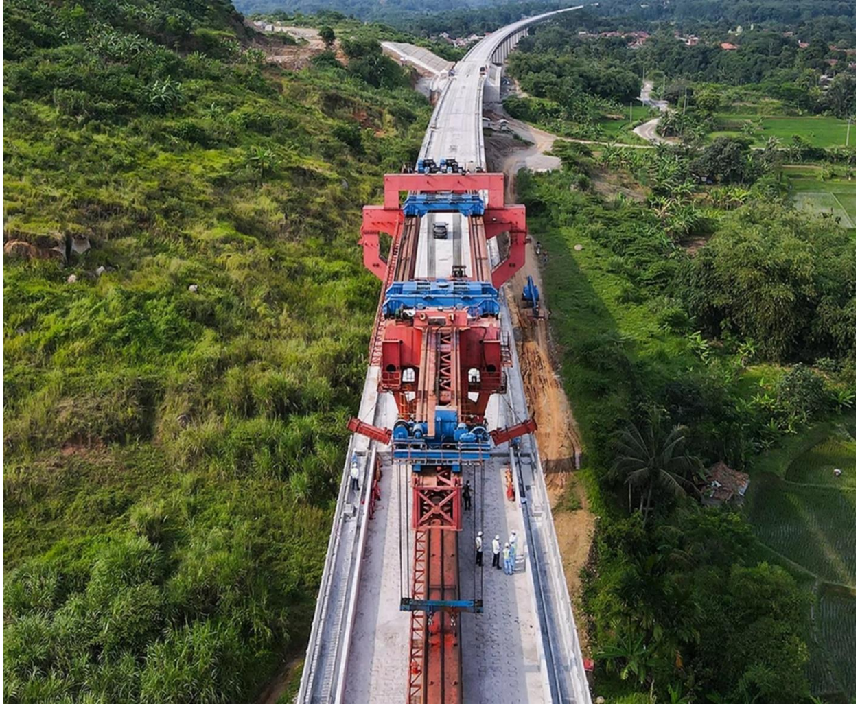
Figure --- Construction of BRI funded railway in Indonesia
