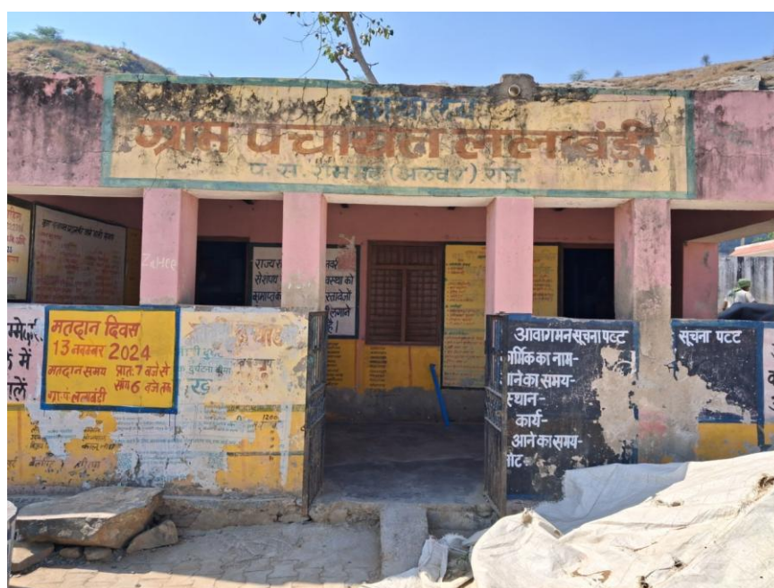
Fig 6.2: Panchayat office of village ‘Lalawandi’
