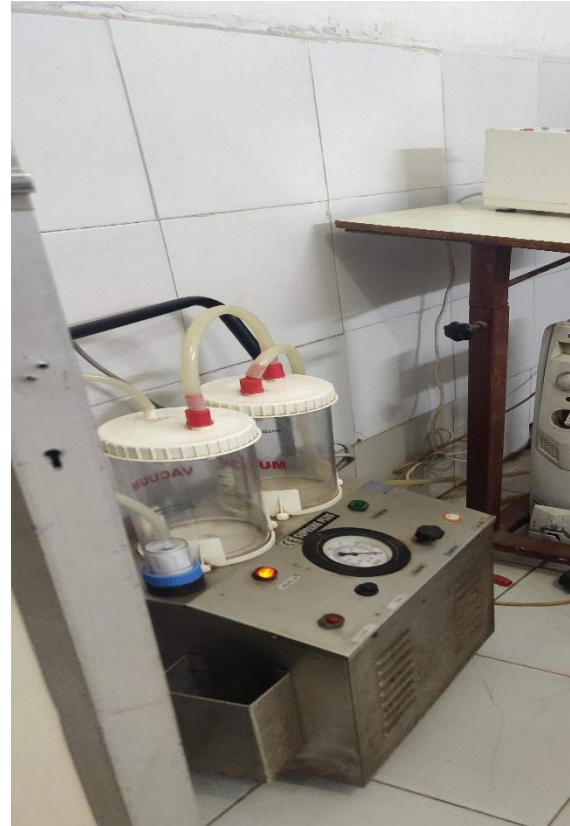
Labour room with suction, heater, Needle destroyer and Newborn Radiant heater
