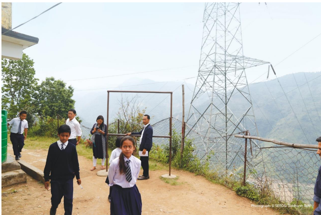
Picture 2.2 High tension wire in close proximity
