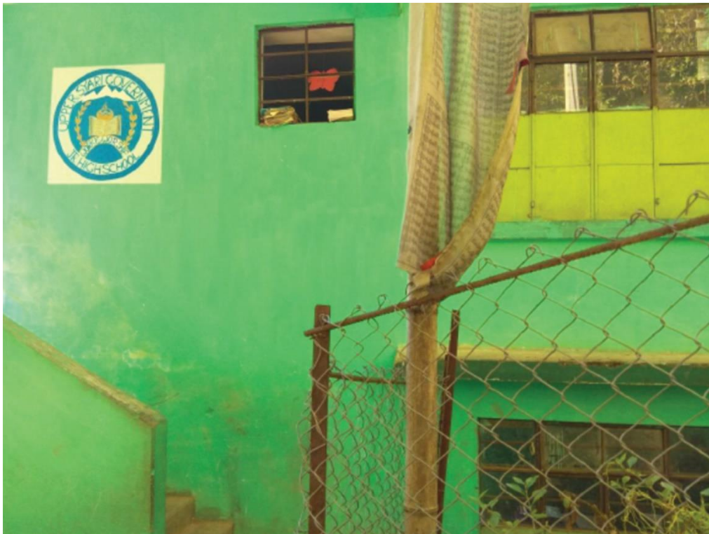
Picture 5.5 Risk Description: cracks in the school building
