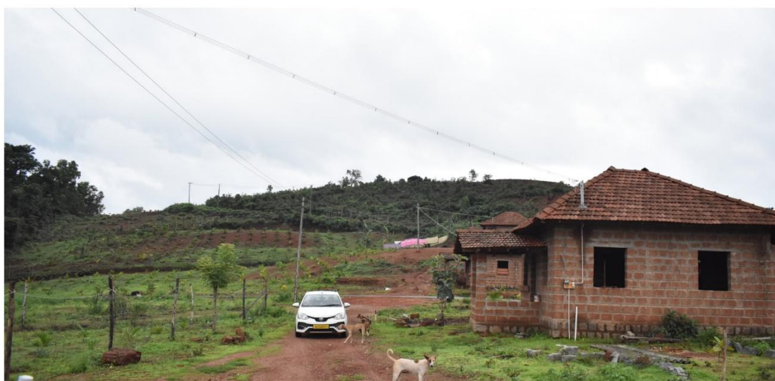
Newly Constructed house for Koraga community in Battuguli under CCDP Funds by ITDP.
