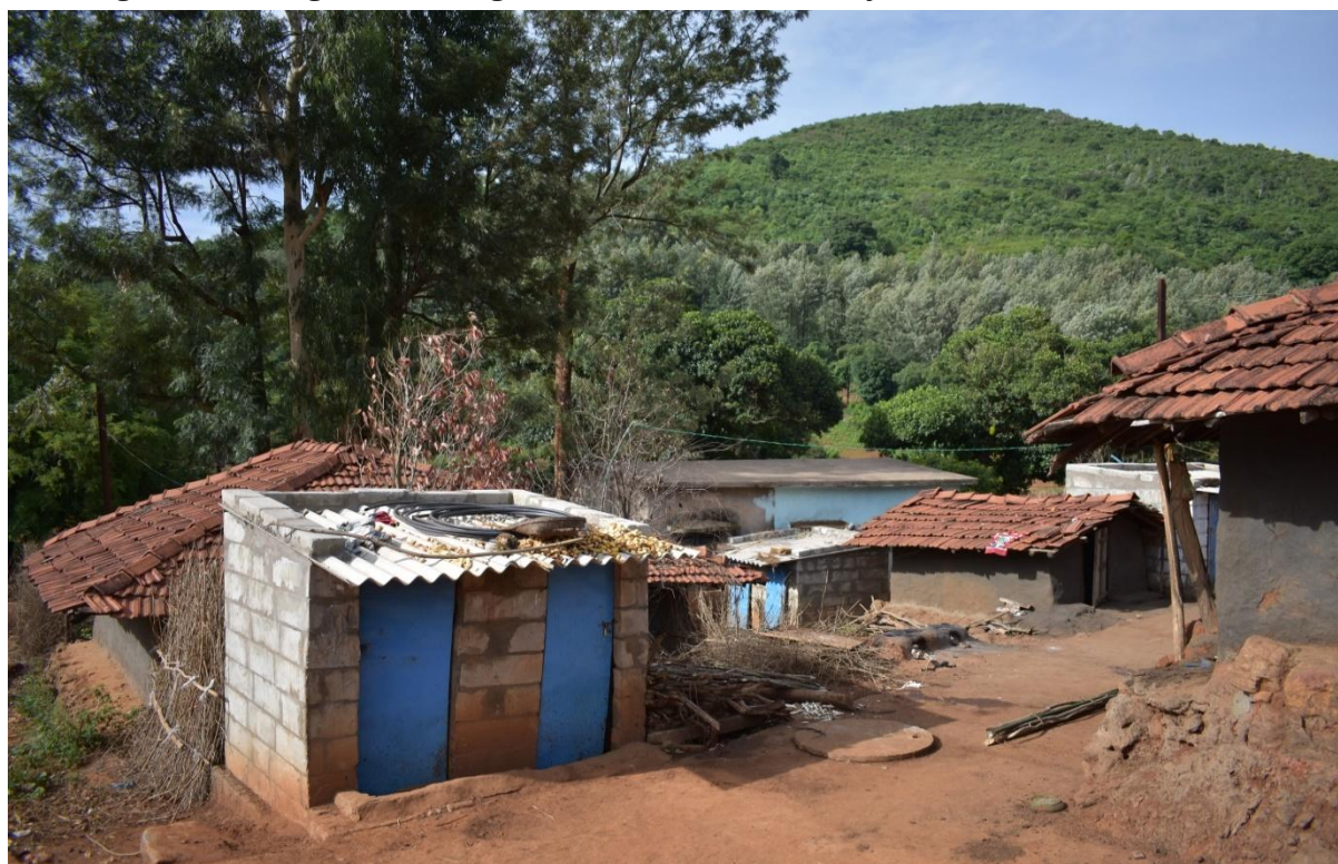
Toilets provided under Swacch Bharat Mission and Semi-pucca houses under IAY in Y. Pedapalli
