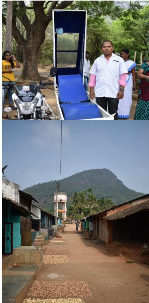
Feeder Bike Ambulance in Sappogothally & CC Road and Over Head water tank in Addamguda, PVTG-Gadaba
