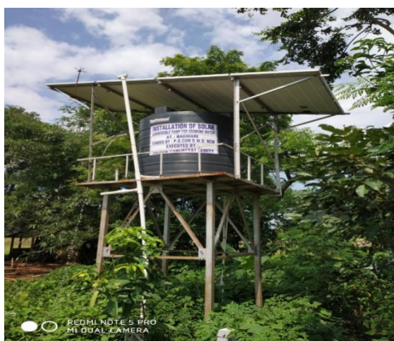
Solar based drinking water system
