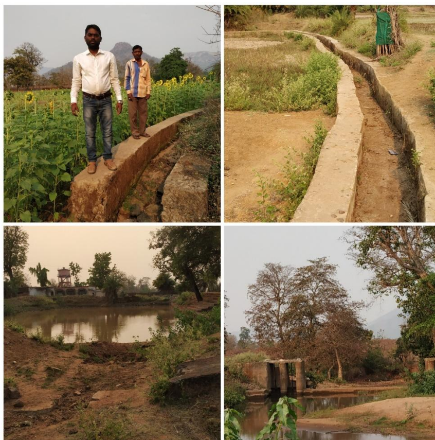
Photographs of Micro Irrigation System constructed by DDA under CCD project.
