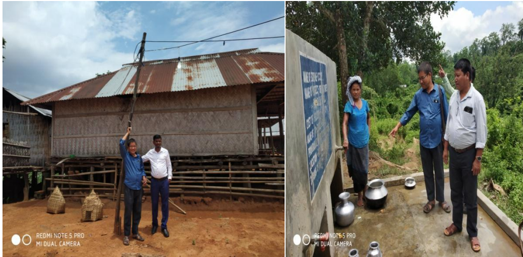
Solar Street Light and Solar Based Drinking Water System
