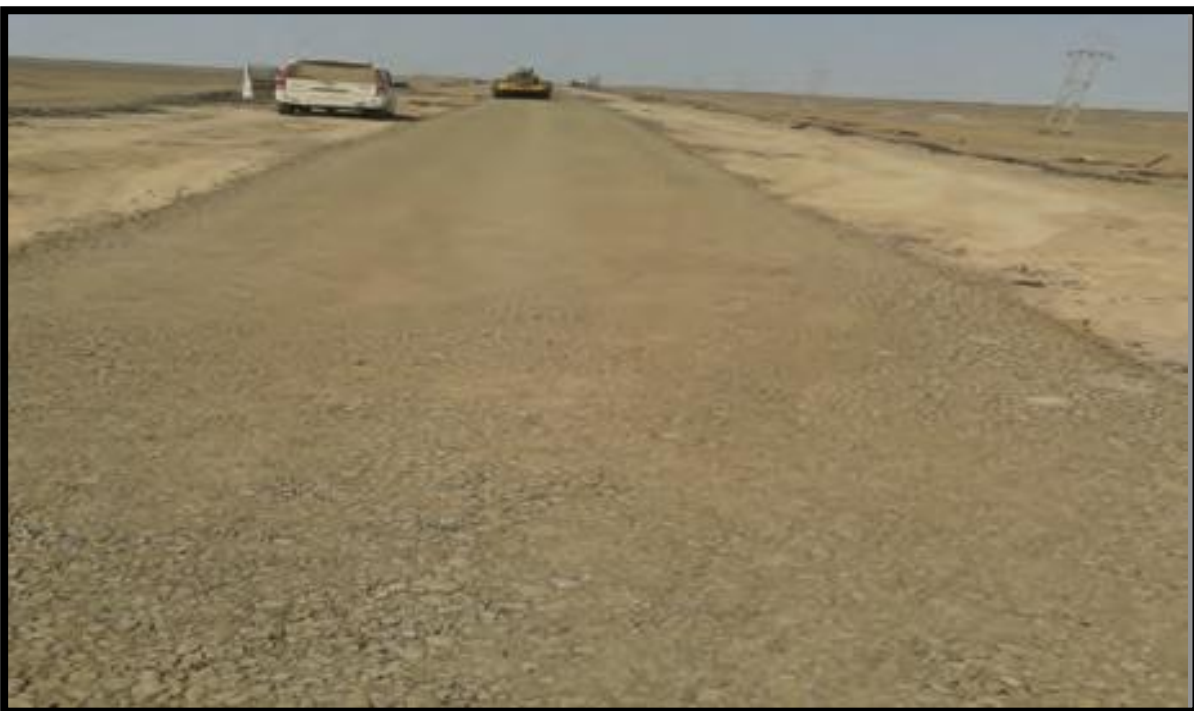
Figure 2.20 Construction of border roads (MHA Annual Report 2015-16)
