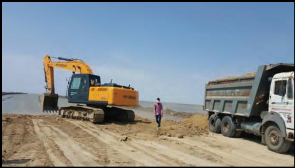
Figure 2.19 Border Road under construction (MHA Annual Report 2015-16)
