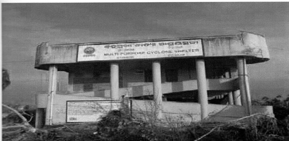
Figure 10: Multi Purpose Cyclone Shelter,Ganjam
